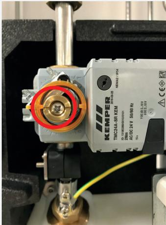
The notch on the spindle is now horizontal.
